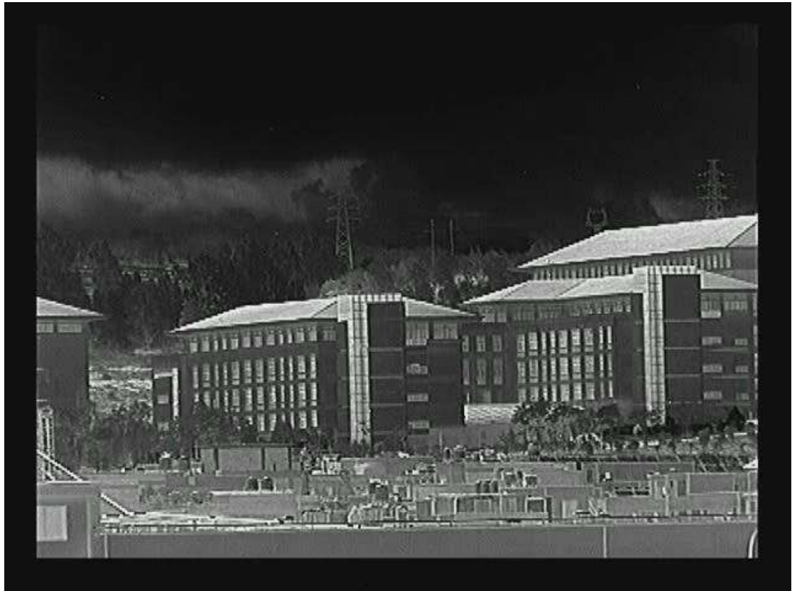
Figure1 Thermal imaging image
